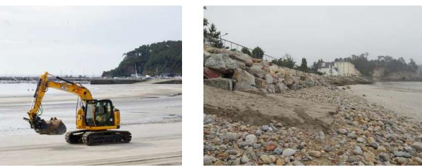
Photo sequence (A–C): Excavator and truck relocating sand due to sediment deficit. After just one tidal cycle, the gravel berm re-emerges, indicating rapid erosion. This operation is repeated every four days.
